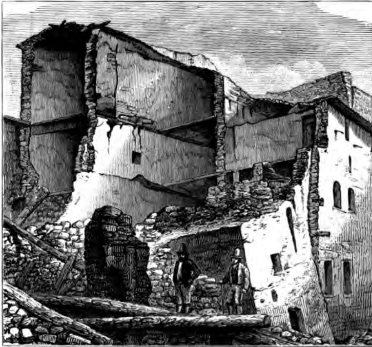
FIG. 113.—STREET VIEW IN LA POLLA AFTER THE EARTHQUAKE OF 1857.
